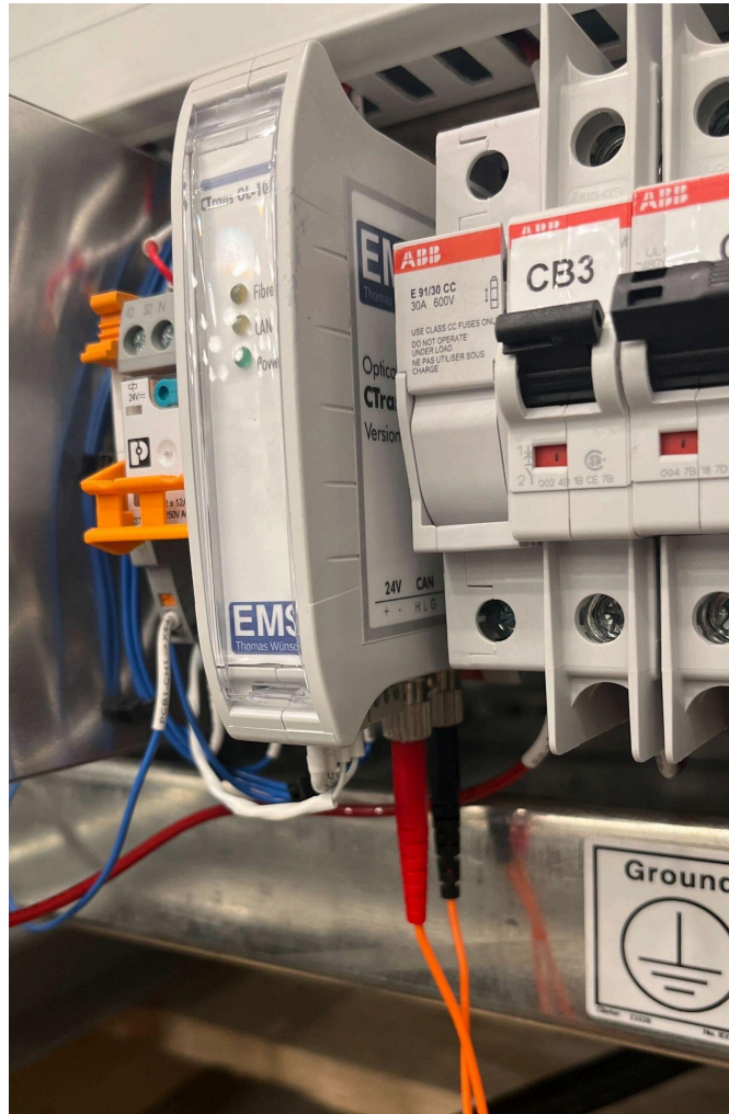
Figure 14. Fiber connection in Power Tower to Charge Cube.
